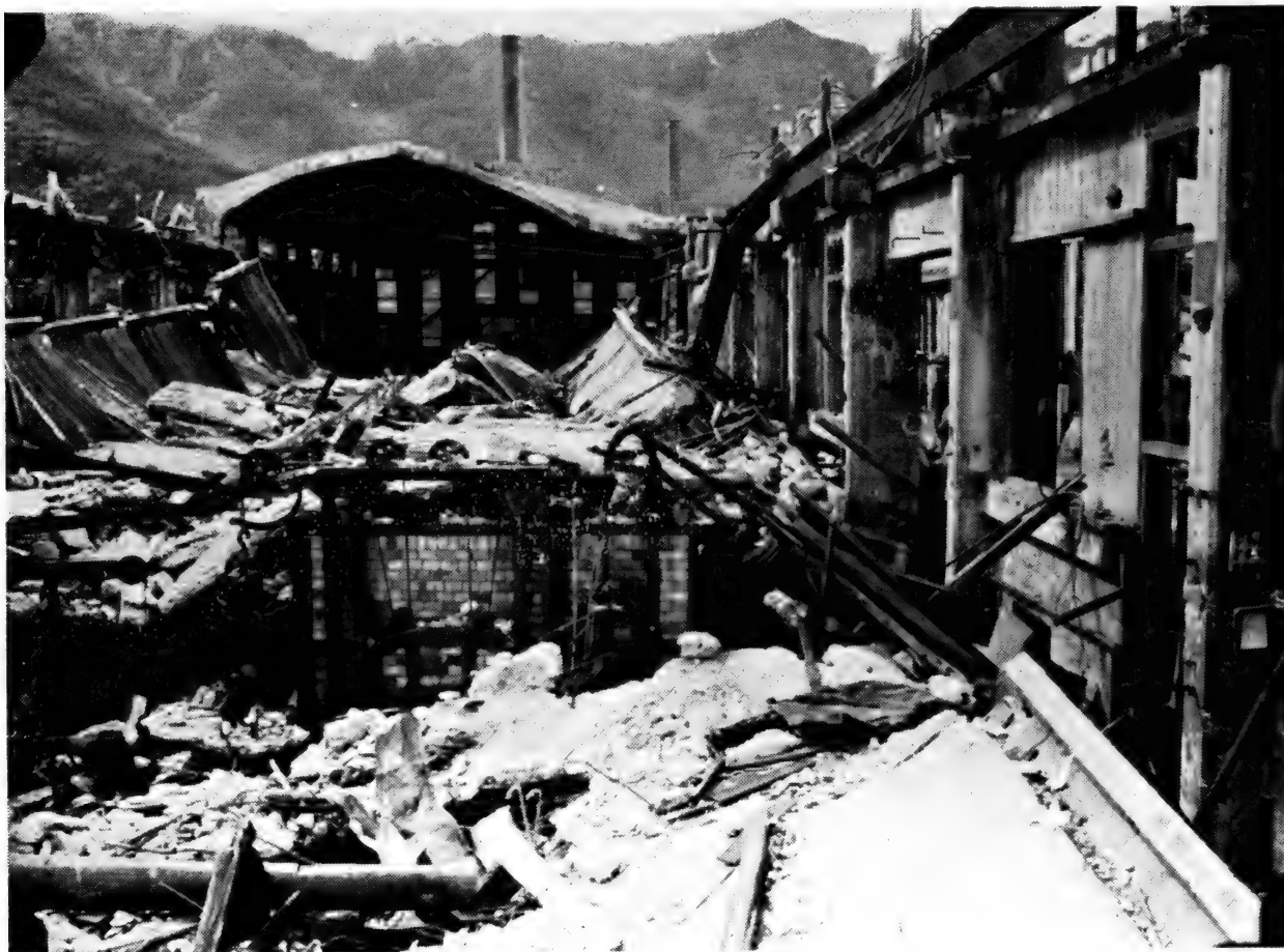
Photo No. 10. NAGASAKI. Reinforced concrete single storey factory rather less than a mile from the centre of damage, which is to the right. The arched reinforced concrete roof failed, the side nearer the explosion being forced inwards and the far side forced upwards. See paragraphs 24 and 29.
